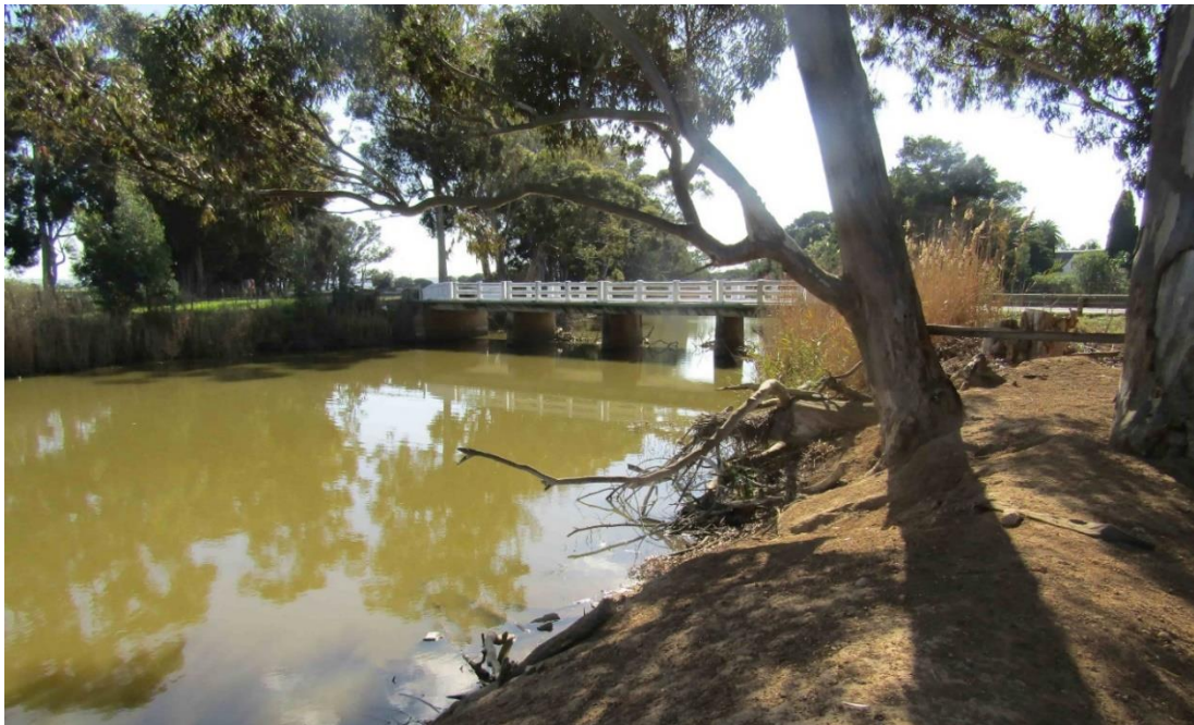
Figure 13. The Kars River under the R316. View to the north.
