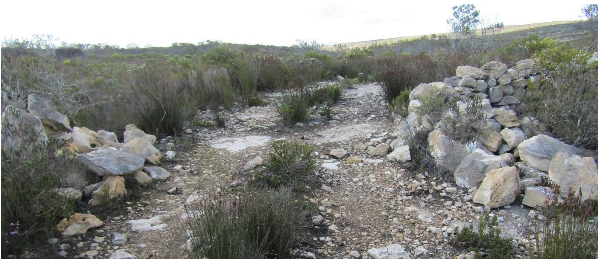
Figure 14. Opening in a stone wall.
