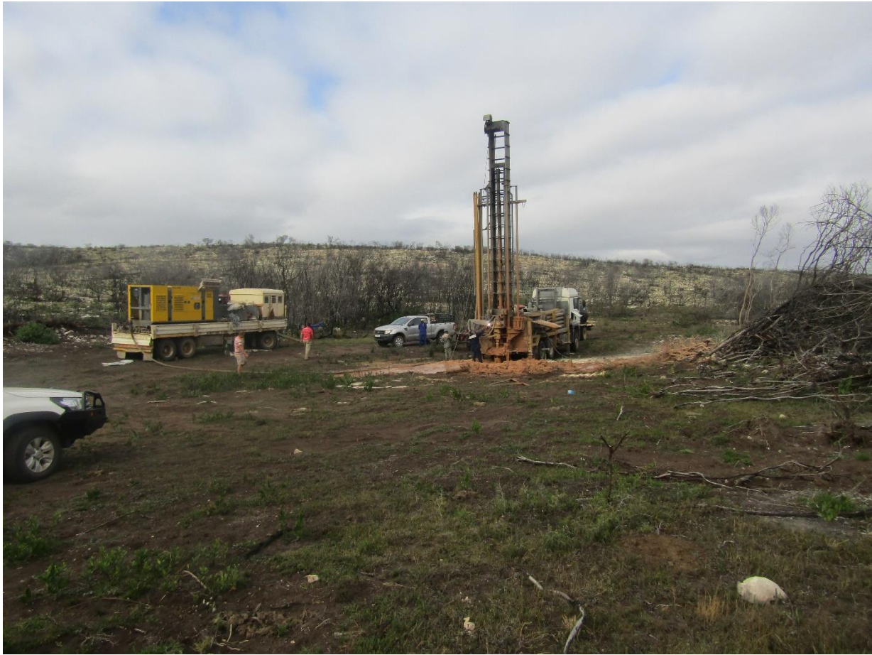
Figure 11. Drilling operations in the southern ravine, Patryskraal Farm. View to the southwest.
