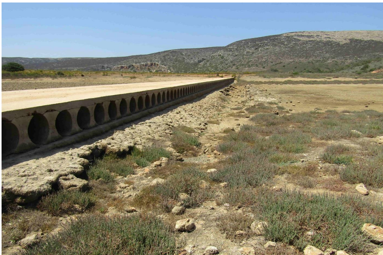
Figure 11. The concrete causeway is about 85 m long. View to the south. The old, rocks causeway can be seen to the right (west) side of the new one. The riverbed is ~8 m above sealevel and the top of the causeway is ~2 m above the riverbed.
