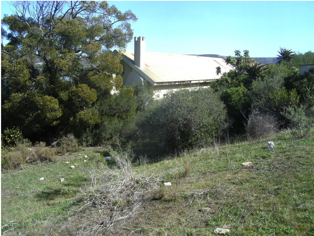
Figure 10. Newer buildings on the historic Windhoek Farm. They were used as offices and staff accommodation of the De Hoop Nature Reserve, some decades ago.
