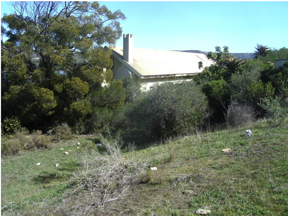
Figure 12. Newer buildings on the historic Windhoek Farm. They were used as offices and staff accommodation of the De Hoop Nature Reserve, some decades ago.
