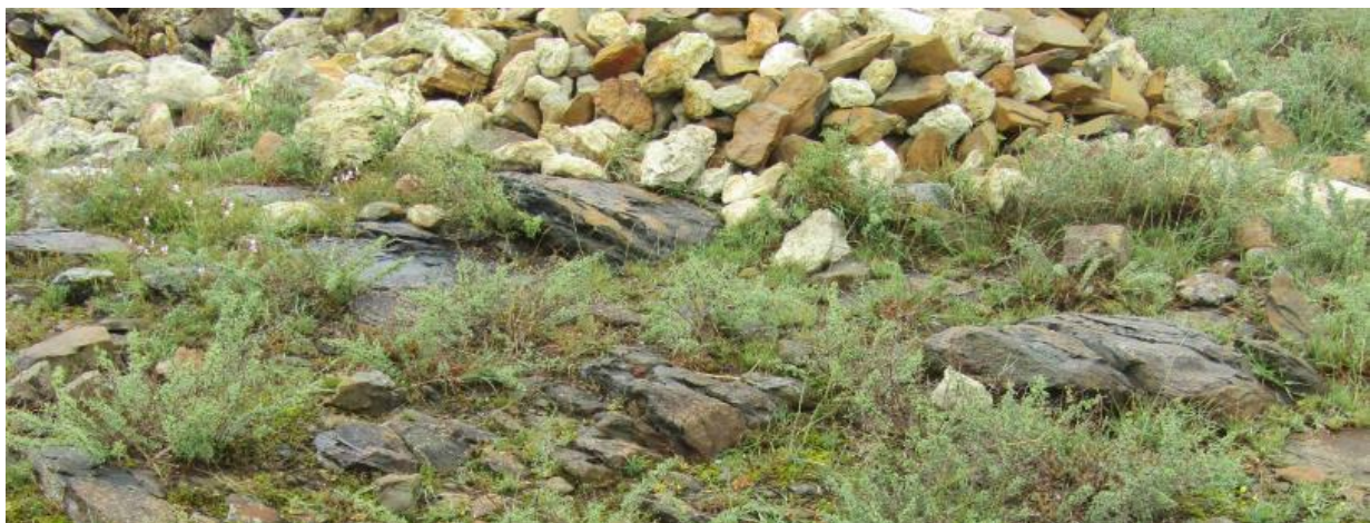
Figure 4. Calcrete on the Ceres Formation. Compact calcrete chunks (top) are heaped on calcrete patches (middle) or on the protruding shales (bottom).
