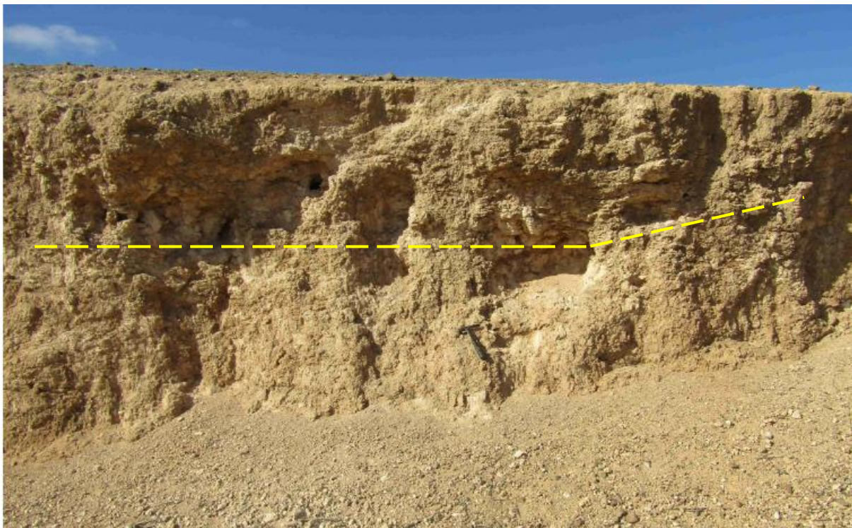
Figure 4. Top and bottom, in a digging, at the heart of the Soutpansvlakte Basin (~1 km east of Patryskraal Farmhouses): Calcrete layer, 1-1.5 m thick over Enon Formation deposits. The dashed line represents the contact between the formations.
