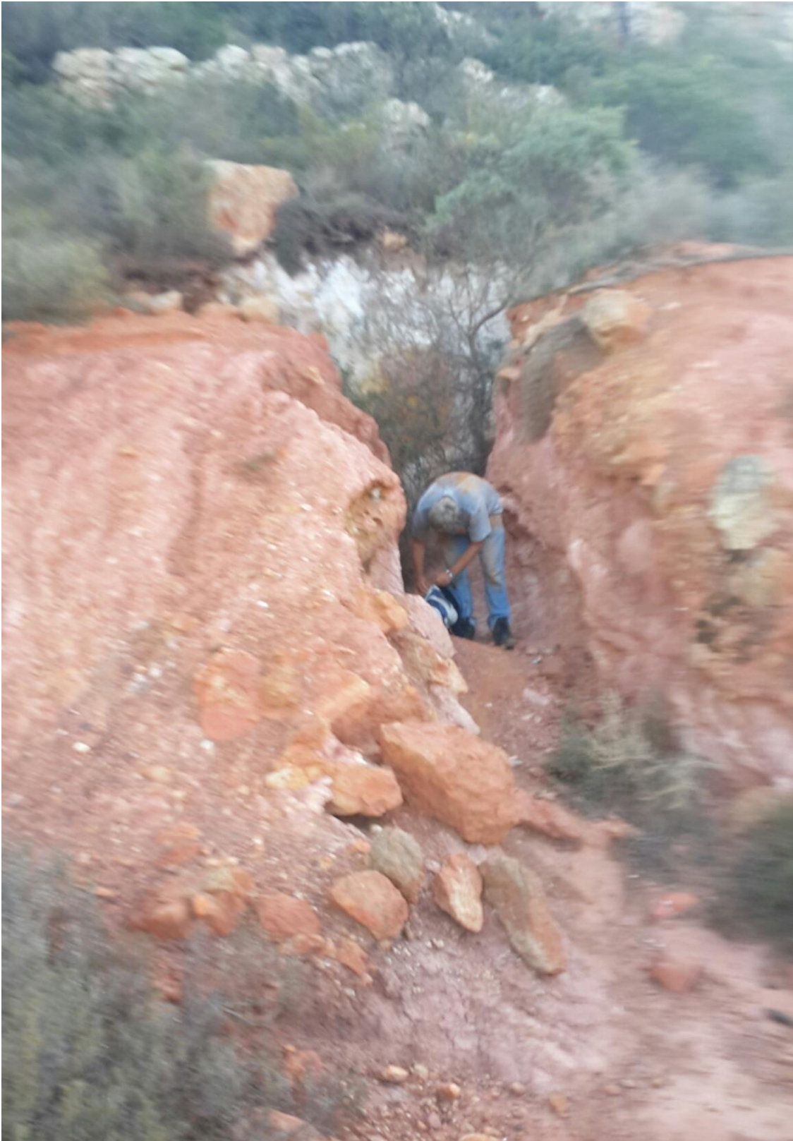
Figure 16. The excavated access to the entrance to one of the two mines on the east side of Hill 288.
