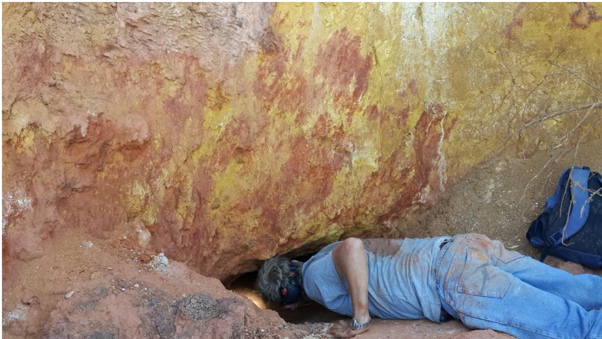
Figure 17. The entrance to the mine on the east side of Hill 288. (The person investigating the underground mine is J Groenewald, of the Renosterveld Research Centre).
