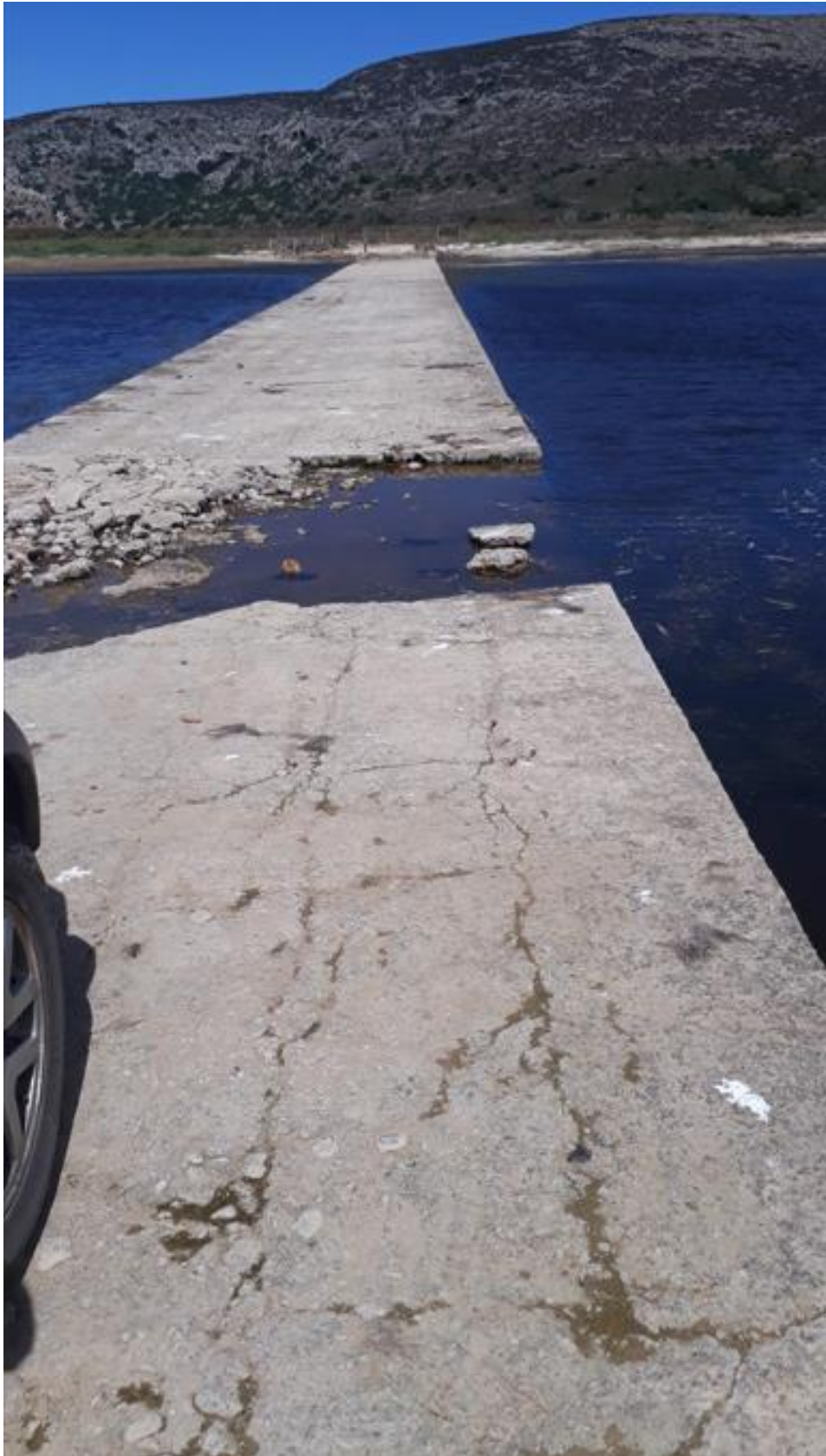
Figure 6. The damaged causeway.
