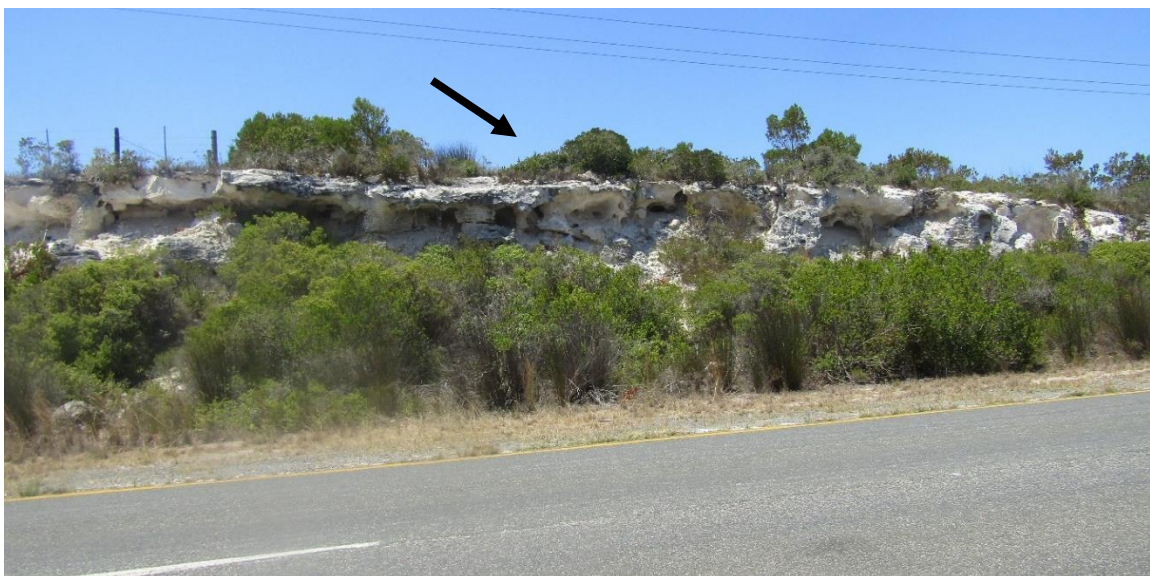
Figure 5. The calcrete hills can attain heights of ~4 m above the surrounding ground, as the one in these photos (arrow), which is crossed by the road from Bredasdorp to Cape Agulhas. Top – geology map; middle – satellite image; bottom – view across the road.
