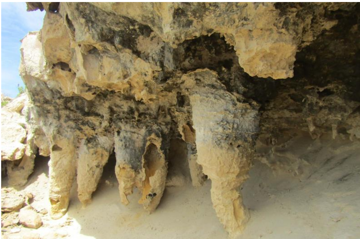
Figure 6. Karst pipes below a calcrete layer (on the North Shore). The yellow box in the top photo indicates the view shown in the bottom photo.
