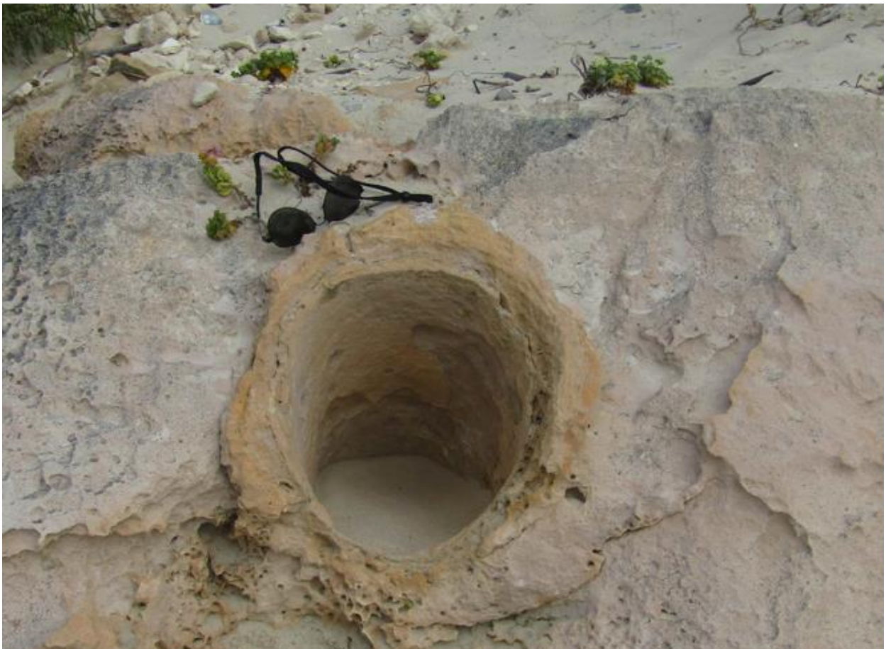
Figure 5. Top and bottom - exposed pipes on the North Shore.
