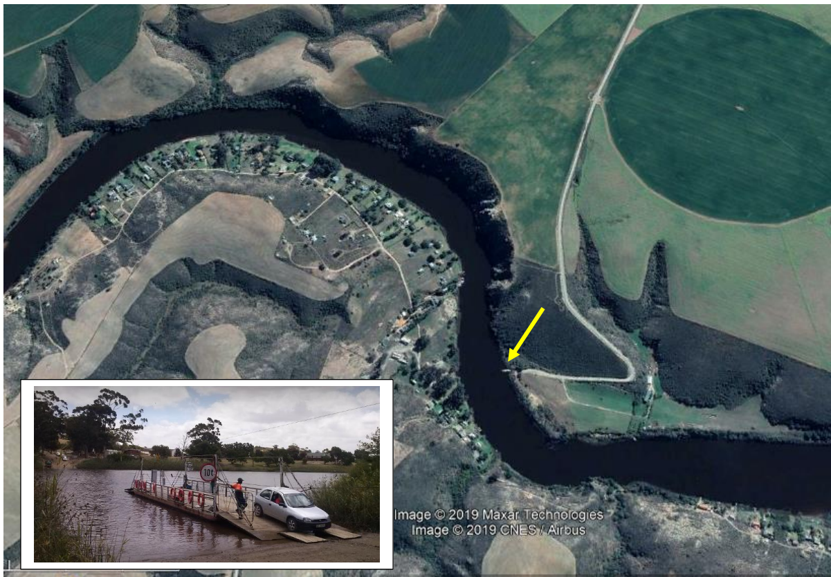
Figure 10. Satellite image of Malgas, where it was possible to cross the Breede River on a hand-pulled pontoon-ferry (arrow and inset). The ferry was replaced by a motorised one in 2021.
