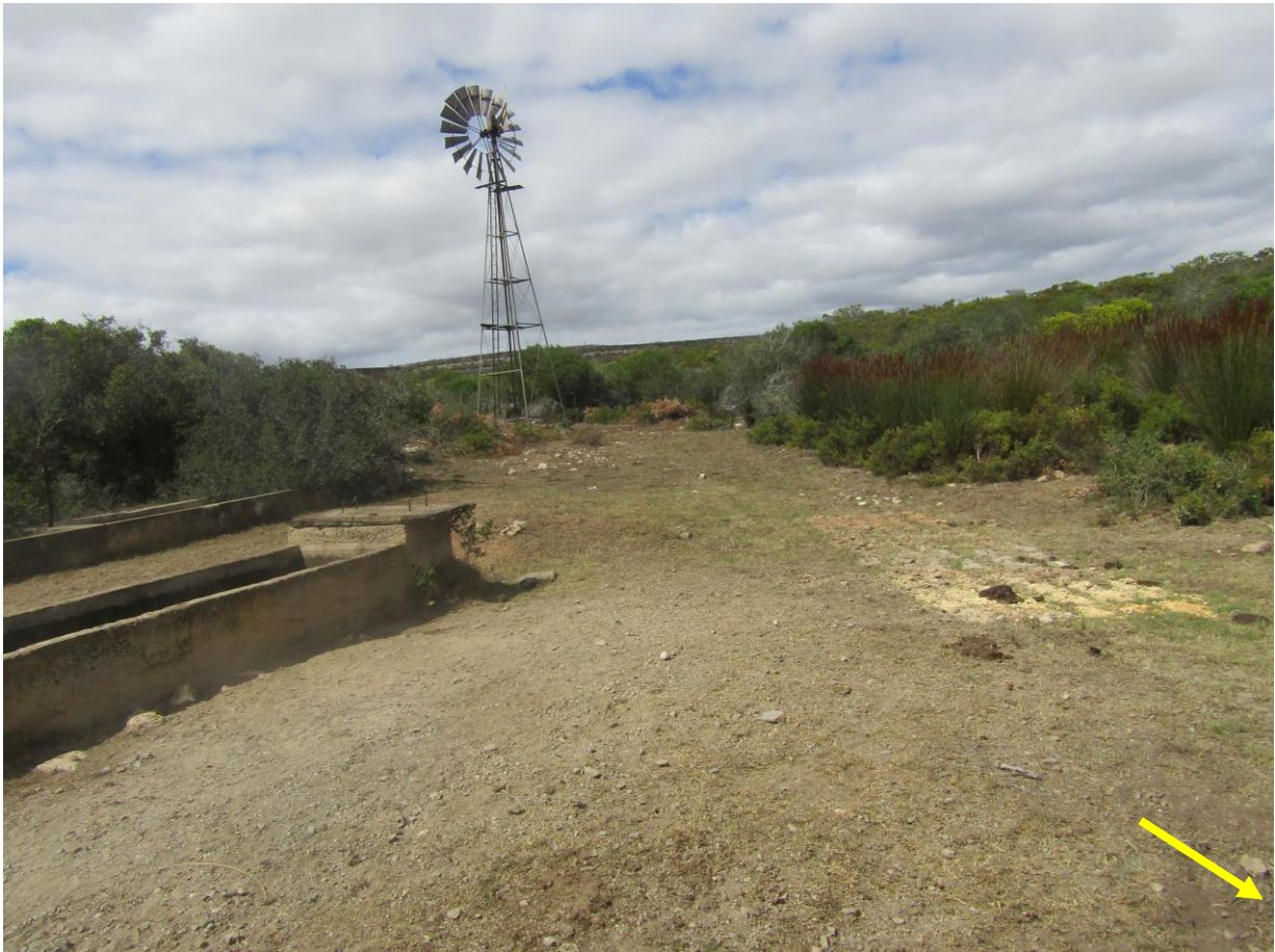
Figure 14. BH 31 and site of new borehole 32 (yellow arrow), in a ravine on the vd Stelskraal Farm. View to the south. The fire which raged in the area in early 2017 spared this ravine.
