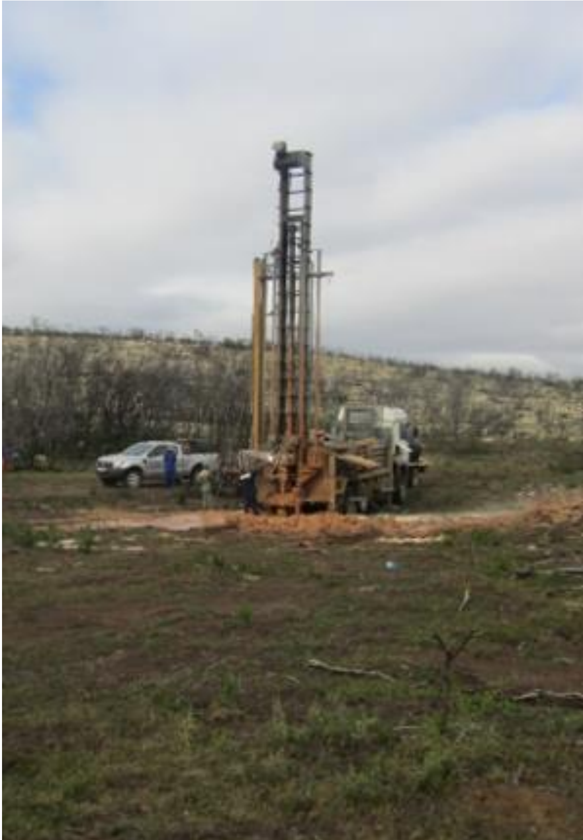
Drilling into the Enon Formation next to the Hard Dunes.
