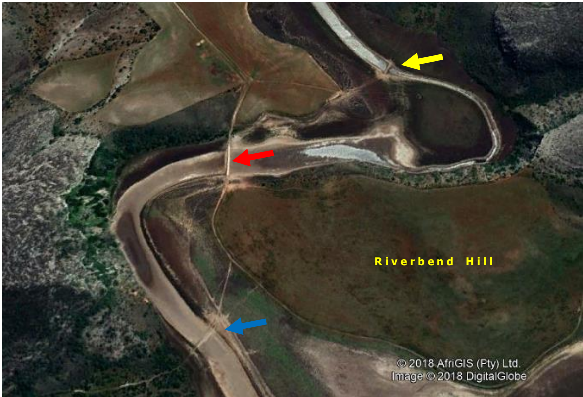
Figure 6. Satellite image of part of the Salt River Gorge from June 2018. The roads and the causeways are exposed.
