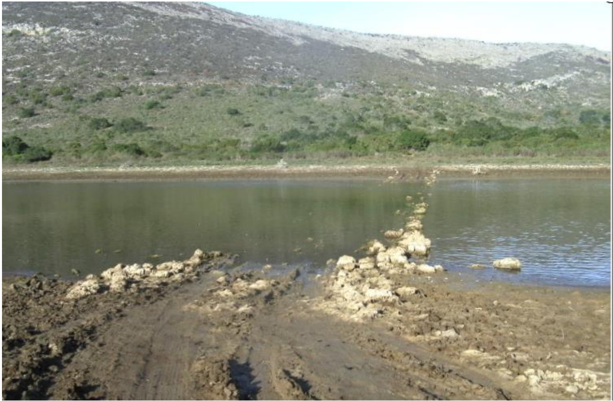
Figure 12. The rocks causeway over the Salt River, leading into Koleskloof, partially submerged. View to the west-southwest.
