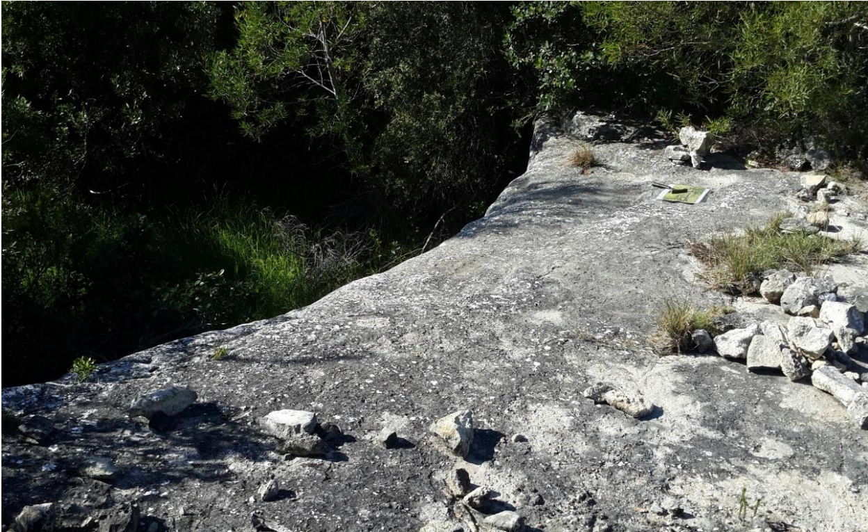
Figure 7. Limestone weir at the bottom of the north wall.
