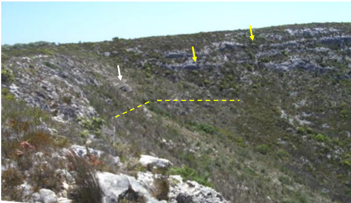
Figure 4. The southwest corner of Koleskloof, view to the north. The nearly right angle between the walls is indicated by a dashed yellow lines. Yellow arrows indicate scarps, which may be of tectonic origin. See Figures 1-5. White arrow points to the rock shown in Figure 5.
