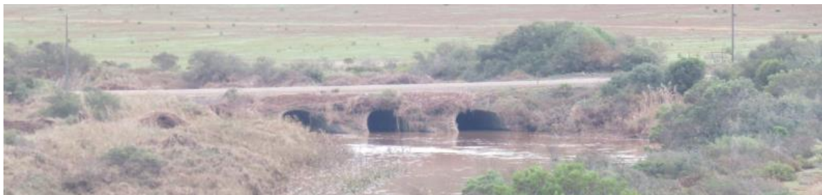
Figure 3. The bridge on the road to Ouplaas. Top – when flooded (arrow points to the bridge); Bottom – after the water receded. The water level is ~1.5 m below the road, or 13 m above msl.
