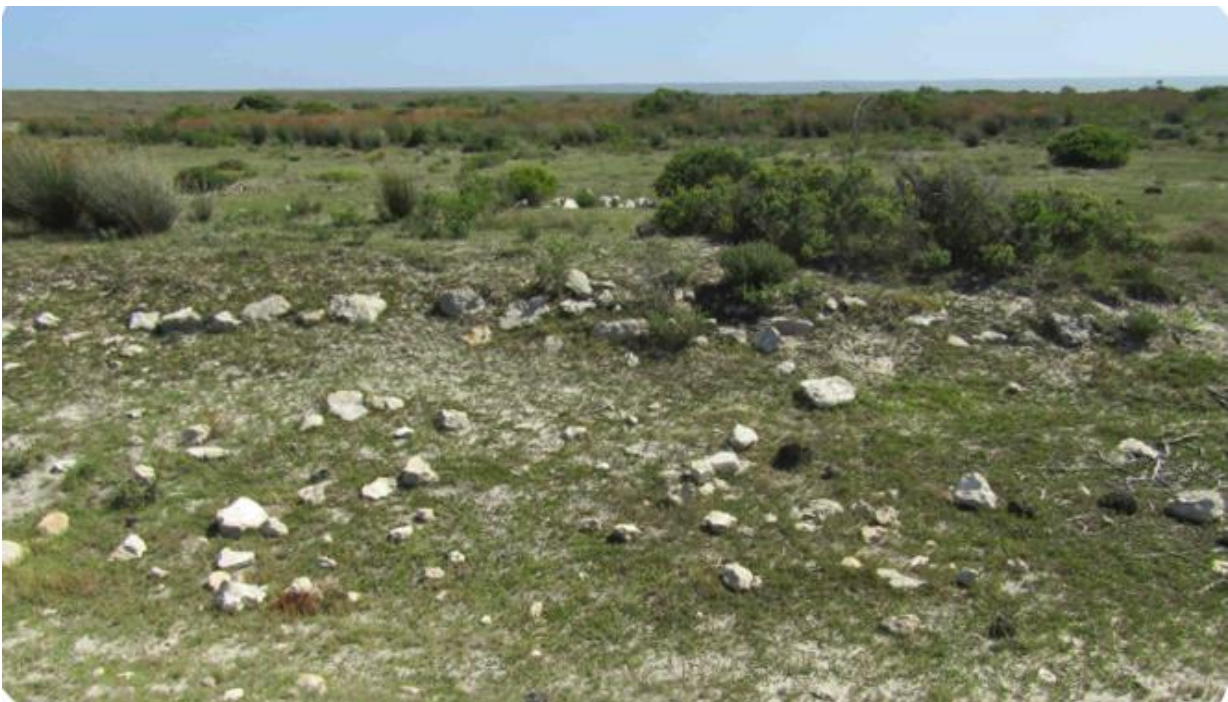
Figure 10. The walls of the canal were cladded with stones, to prevent erosion. The cladding disintegrated with time.
