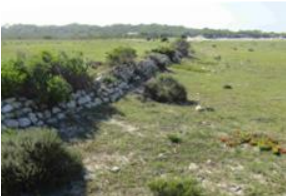
Figure 15. The dyke was cladded on the west (vlei) side. View to the east. The depression is on the left, the vlei on the right.
