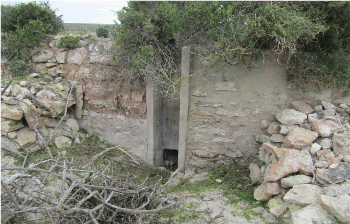
Figure 16. The vlei side of the gate in the dyke.
