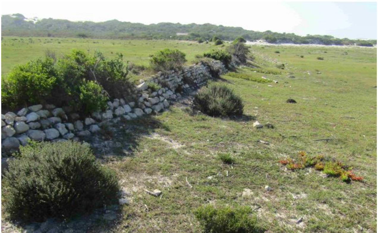
Figure 15. The dyke was cladded on the west (vlei) side. View to the east. The depression is on the left, the vlei on the right.
