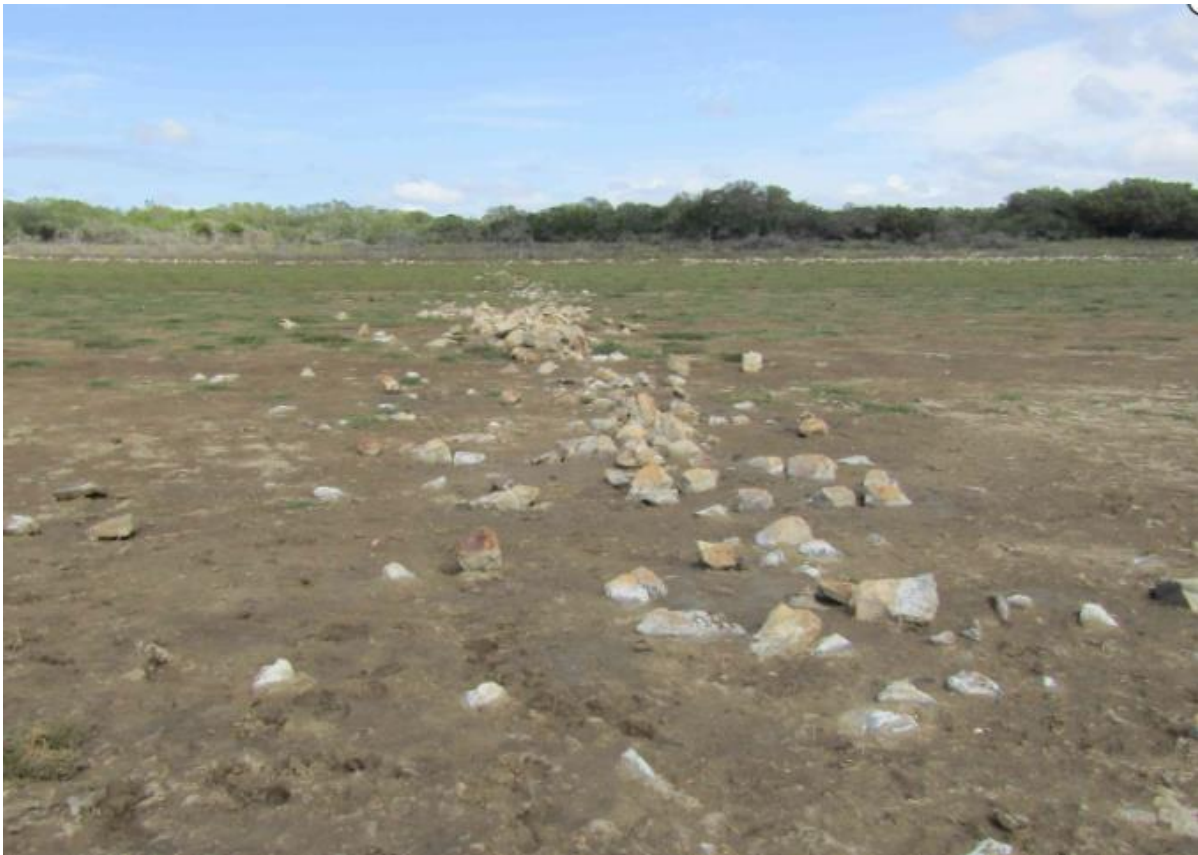
Figure 14. Top - the stonewall along the west bank of the vlei. Bottom - the ruins of the stonewall, which extends into the vlei, from the wall shown in the top photographs.
