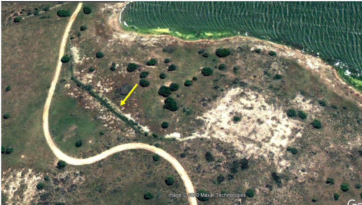
Figure 24. Satellite image of the southern road-protection dyke (arrow).
