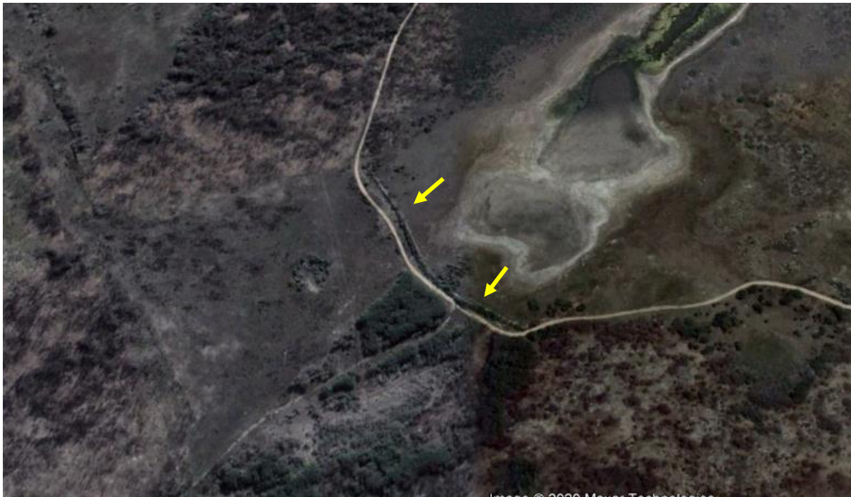
Figure 22. Satellite image of the northern road-protection dyke (arrows).
